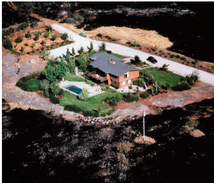
The pre-fire activities implemented by this homeowner included a green and well maintained landscape, reduction of wildland vegetation around the perimeter of the property, a fire resistant roof, and a good access road with a turnaround area. The charred surroundings of the home show that these pre-fire activities effectively protected it when wildfire hit.
